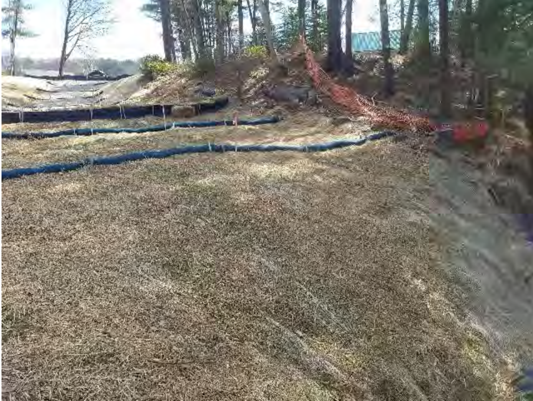
Fig 7: BMPs on slope at Gundalow landing. Viewing south. (04-17-20).
