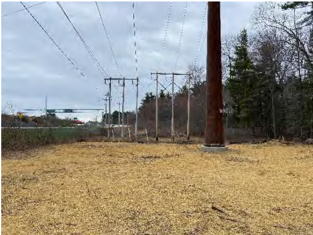
Fig 26: Timber mats removed from Str. 130. Viewing southeast. (04-21-20).
