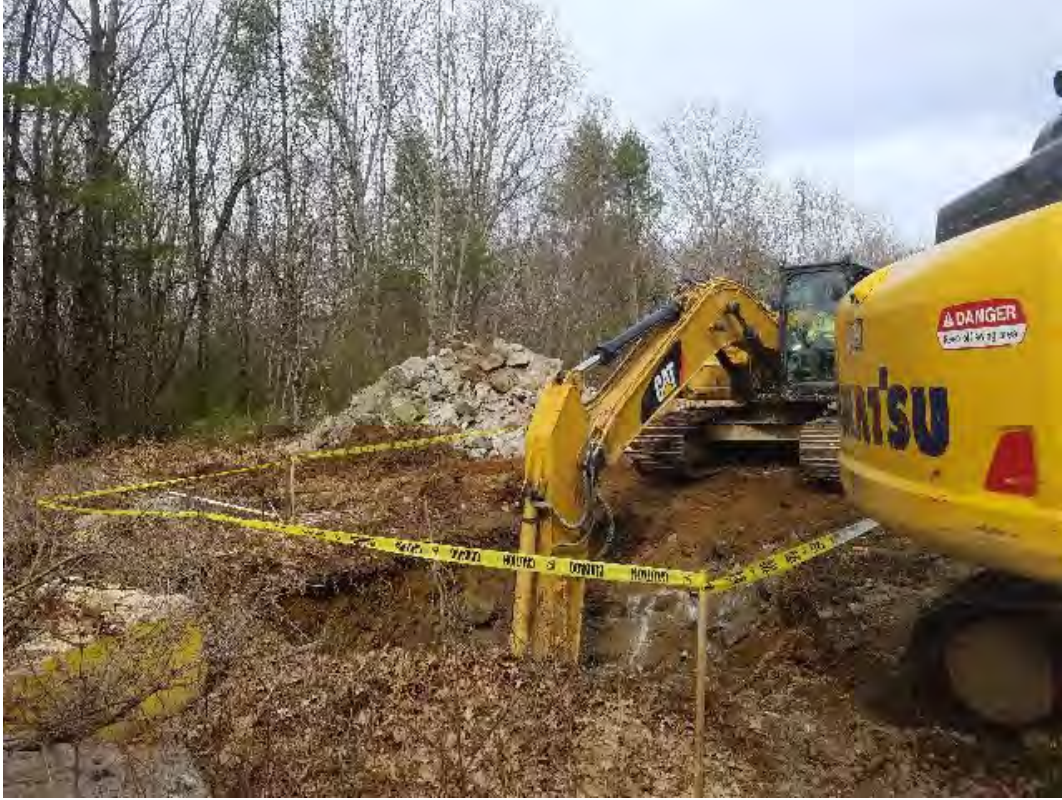
Fig 17: Excavating foundation for Str. 88. Viewing northwest. (04-20-20).
