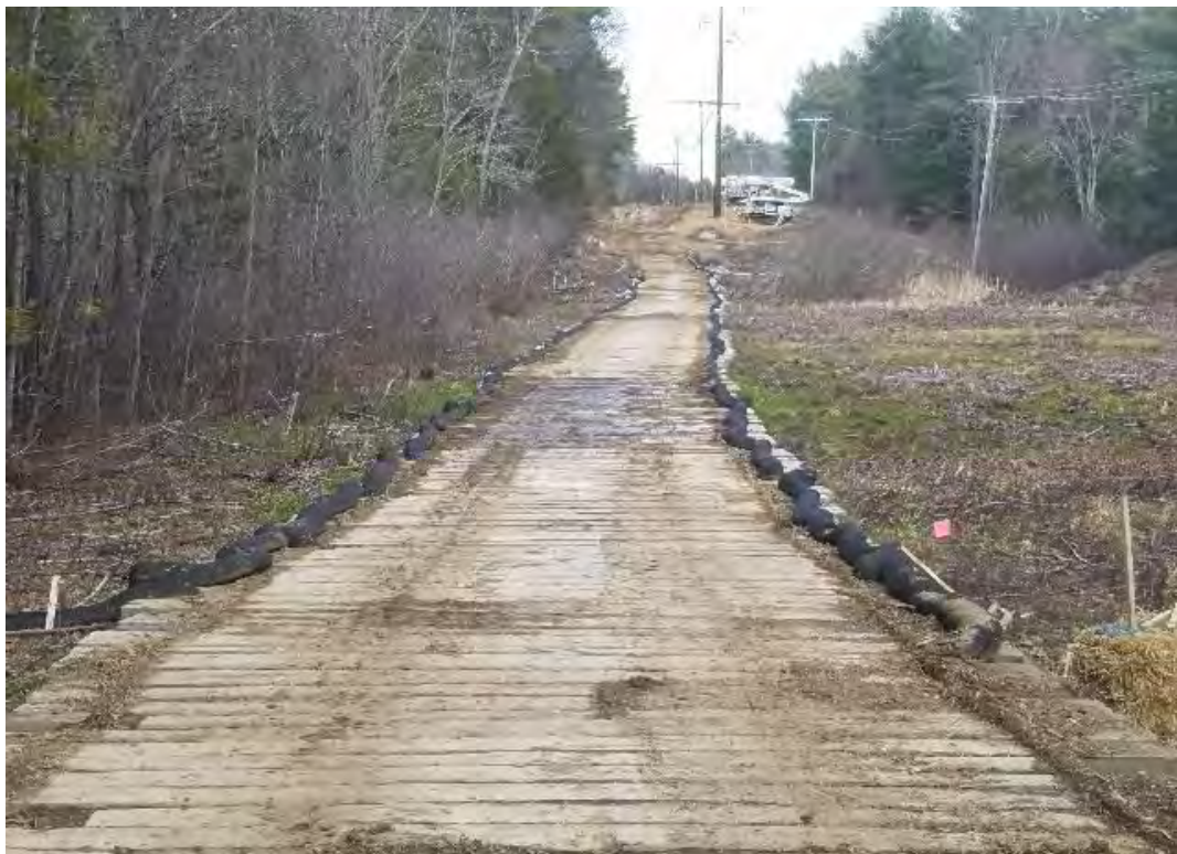
Fig 30: Crews cleaned timber matted access road between Strs. 54 and 55. Viewing northeast. (04-22-20).
