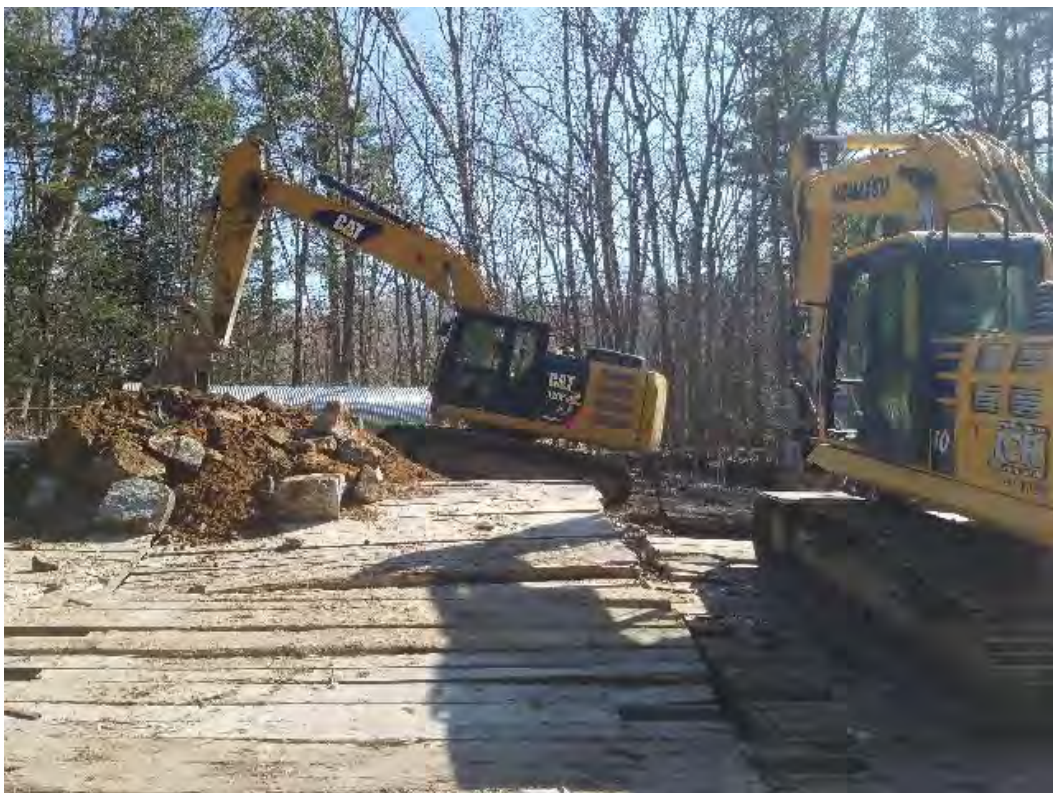
Fig 22: Excavating foundation for Str. 90. Viewing north. (04-21-20).
