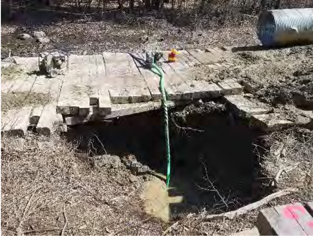
Fig 23: Pumping groundwater from Str. 89 foundation hole. Viewing north. (04-21-20).
