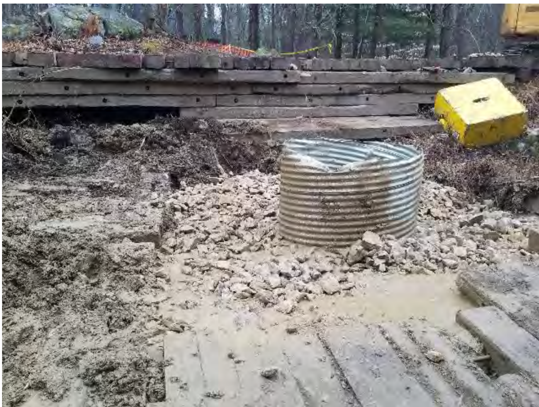
Fig 24: Setting foundation can for Str. 89. Viewing south. (04-21-20).
