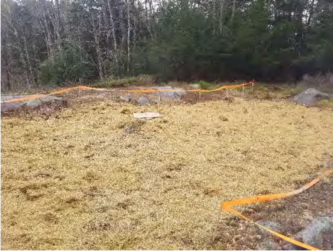
Fig 9: Str. 81 foundation can set. Viewing south. (04-17-20).
