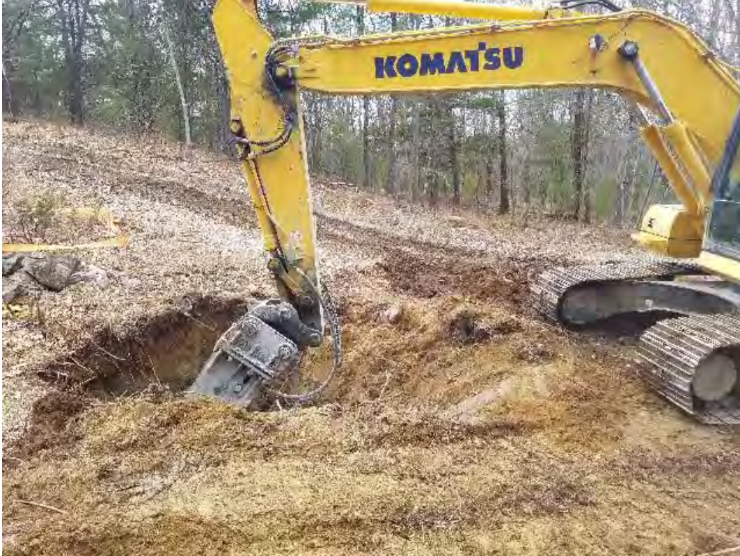
Fig 11: Hammering ledge for foundation at Str. 86. Viewing south. (04-17-20).
