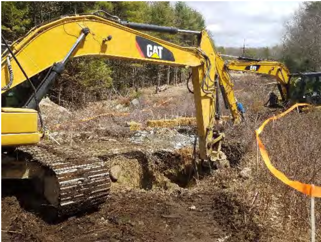
Fig 28: Excavating foundation for Str. 83. Viewing northeast. (04-22-20).
