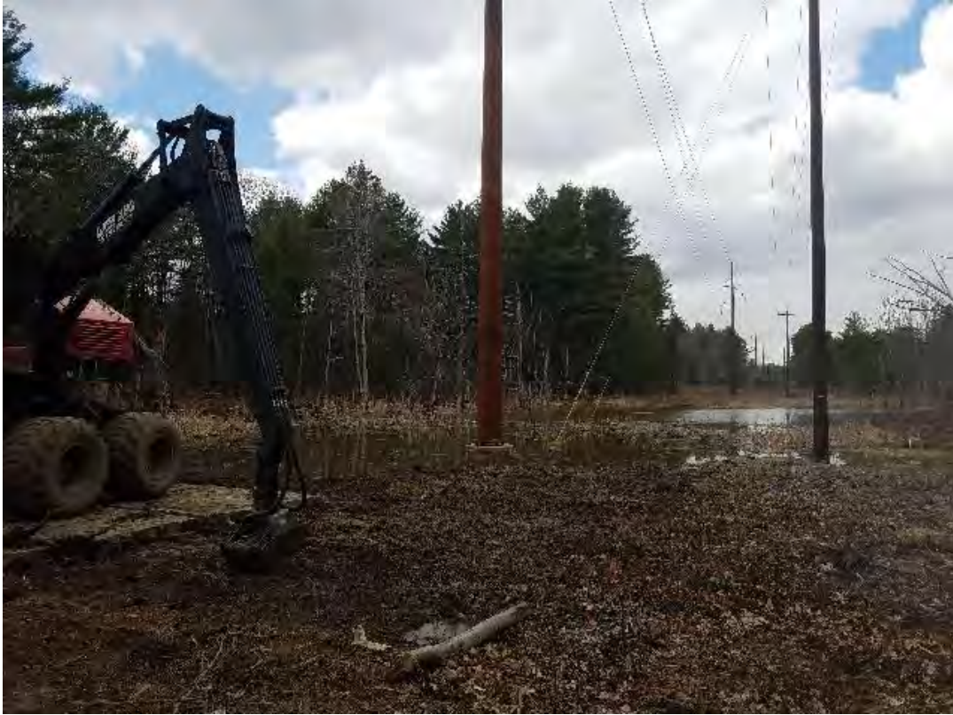
Fig 1: Removing timber mats from access road around Str. 116. Viewing northwest. (04-16-20).
