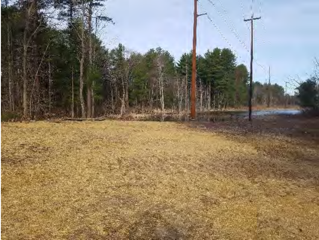
Fig 15: Str. 116 work area after timber mats have been removed. Viewing west. (04-20-20).
