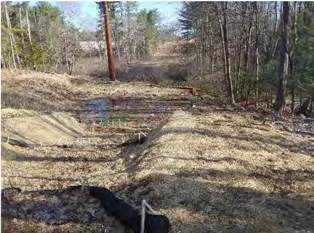
Fig 2: Access to Str. 28. Viewing north. (04-16-20).
