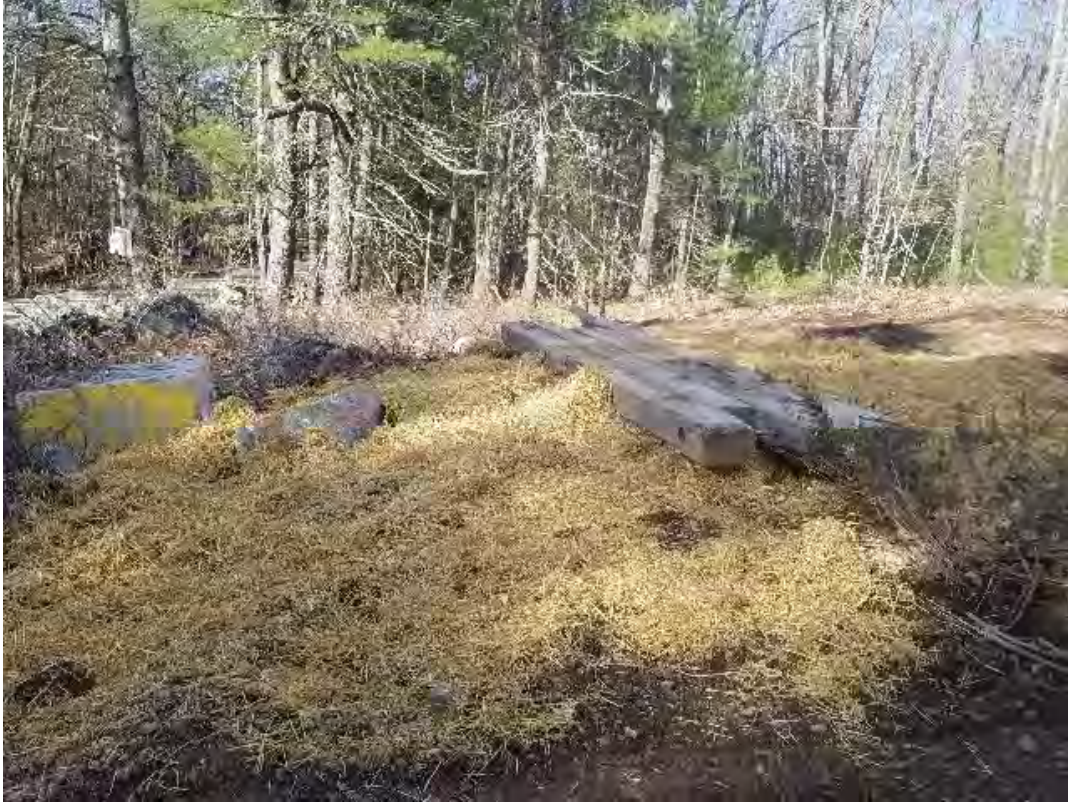
Fig 21: Foundation can set for Str. 88. Viewing west. (04-21-20).
