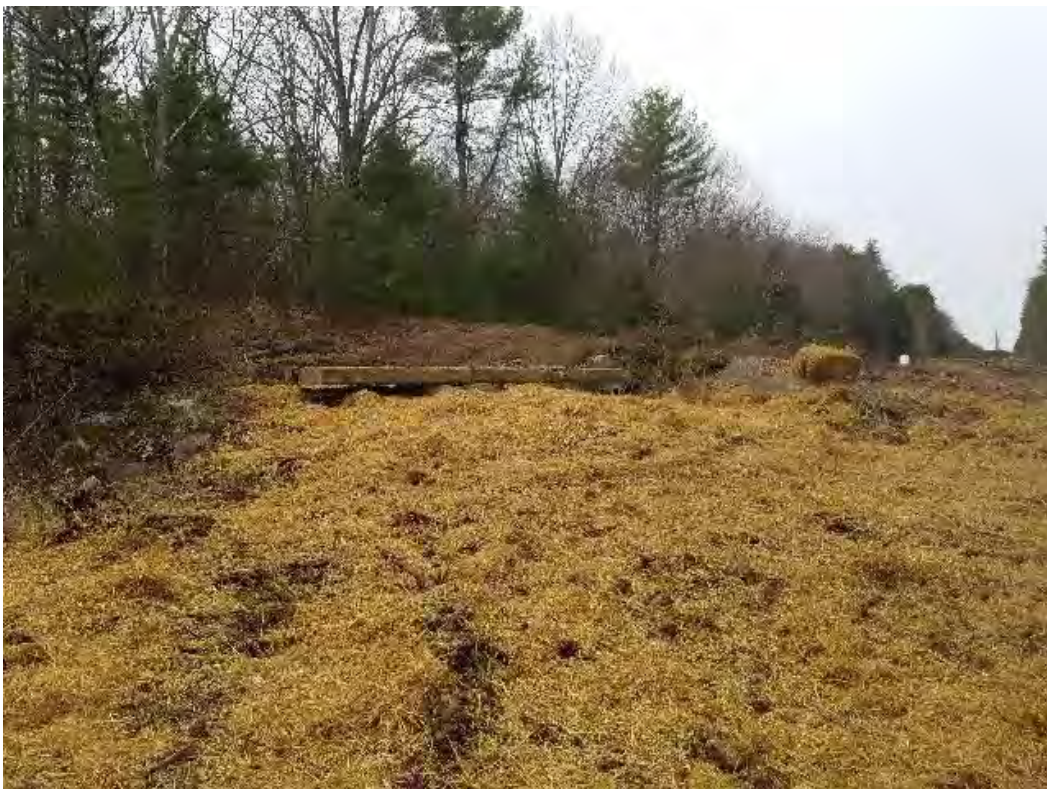
Fig 16: Str. 86 foundation can set. Viewing south. (04-20-20).
