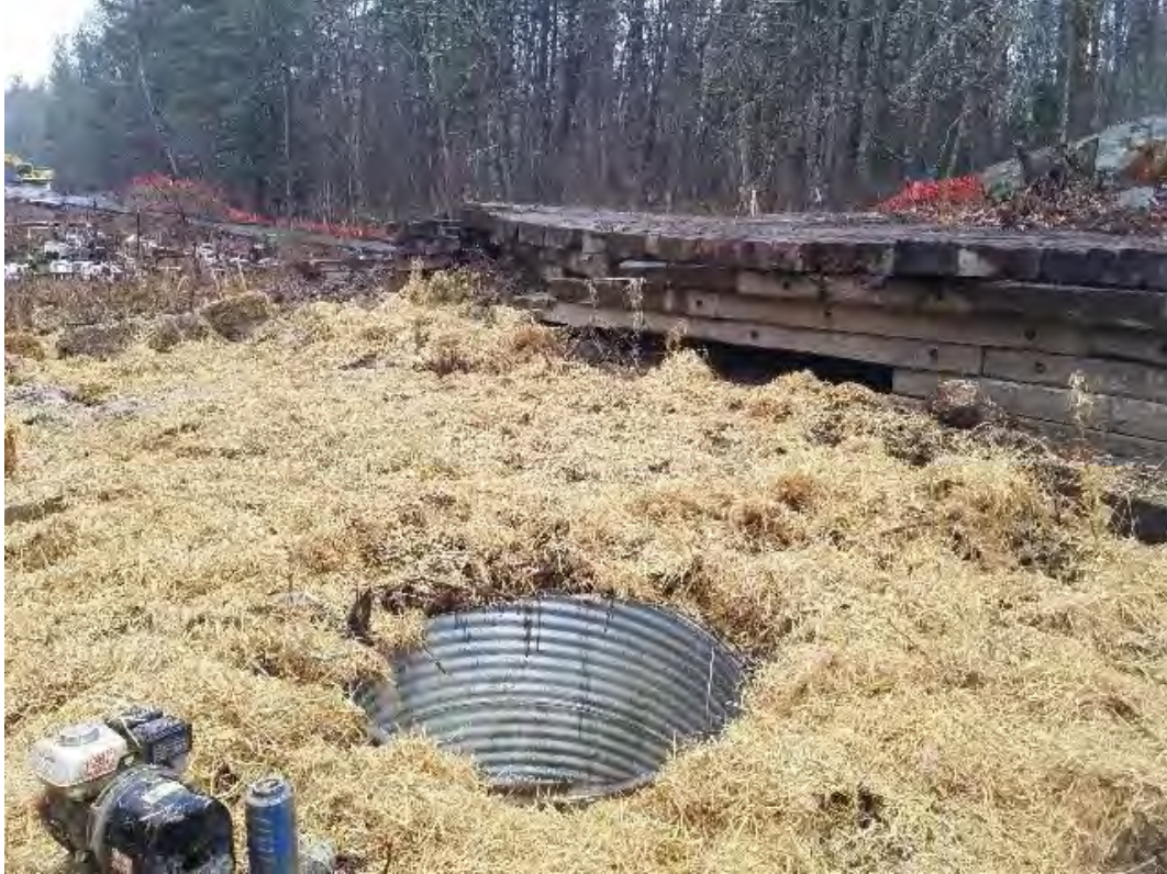
Fig 25: Foundation can set for Str. 89. Viewing south. (04-21-20).
