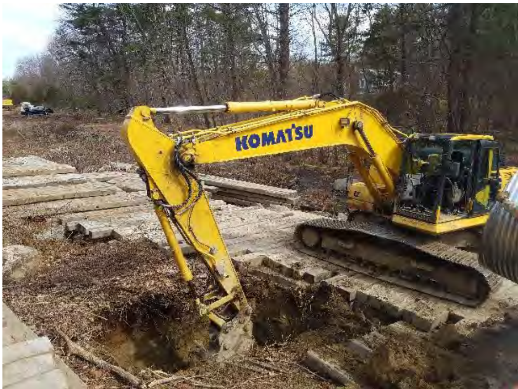
Fig 18: Excavating foundation for Str. 89. Viewing north. (04-20-20).
