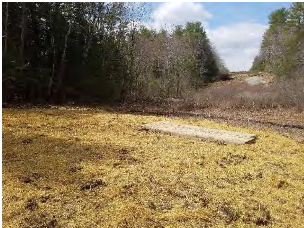
Fig 8: Str. 82 foundation can set (under timbermat – typical). Viewing west. (04-17-20).
