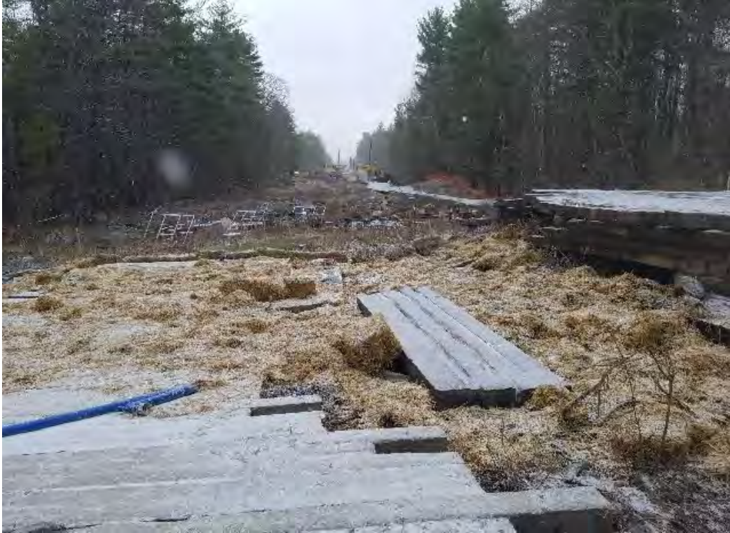
Fig 27: Str. 89 work area. Viewing southeast. (04-22-20).
