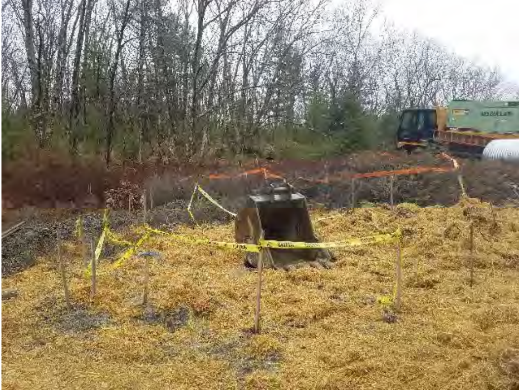
Fig 13: Str. 80 work area. Foundation can not set yet. Viewing southwest. (04-18-20).
