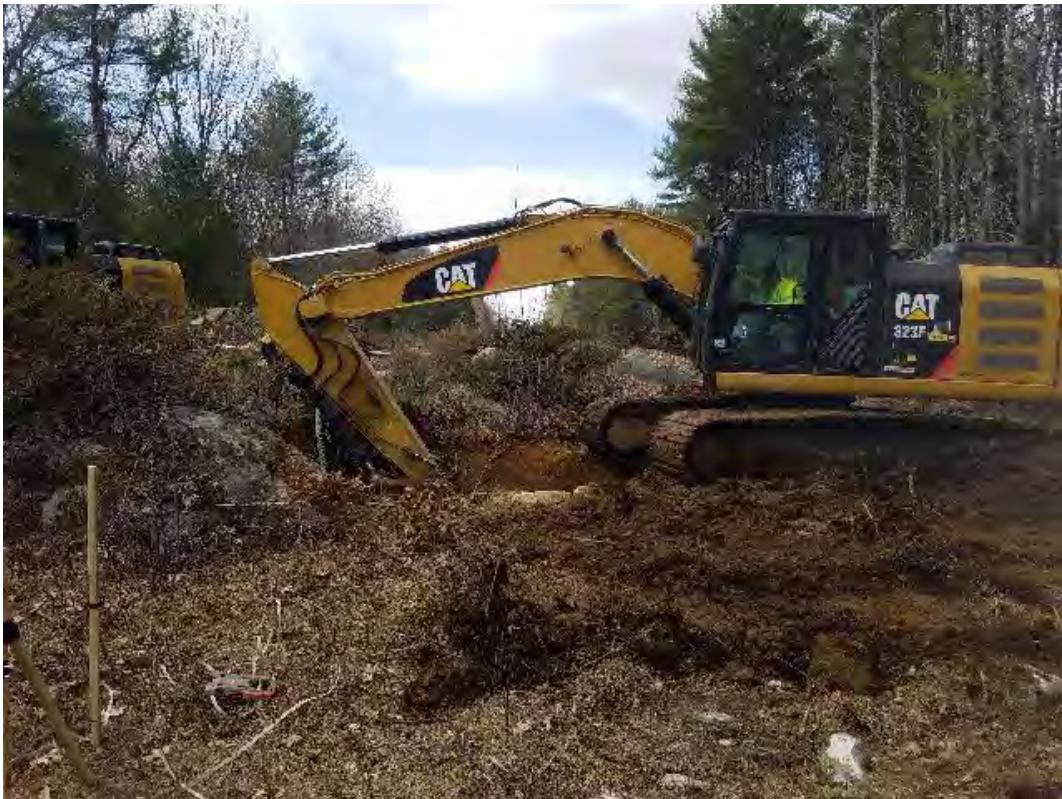
Fig 10: Excavating foundation for Str. 84. Viewing west. (04-17-20).
